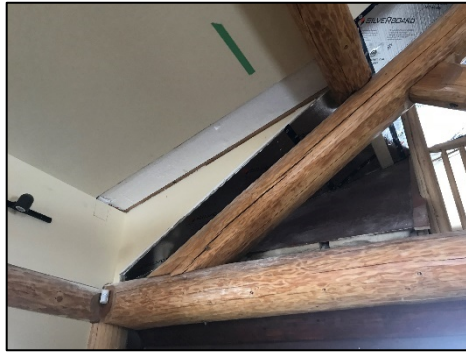
Photo #6: Framing and insulation at roof slope transition
