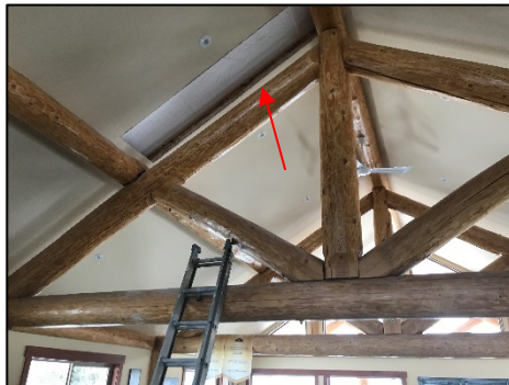
Photo #4: Open ceiling drywall
