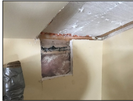
Photo #7: Ceiling to wall junction
