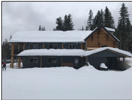
Photo #1: East Elevation
