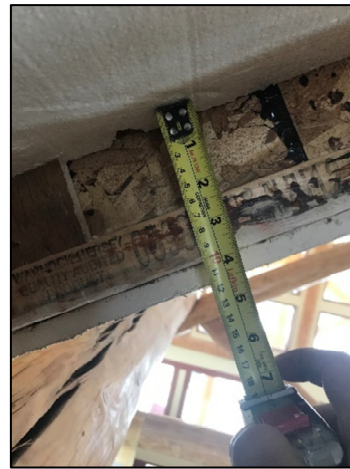
Photo #5: Insulation recessed between joists
